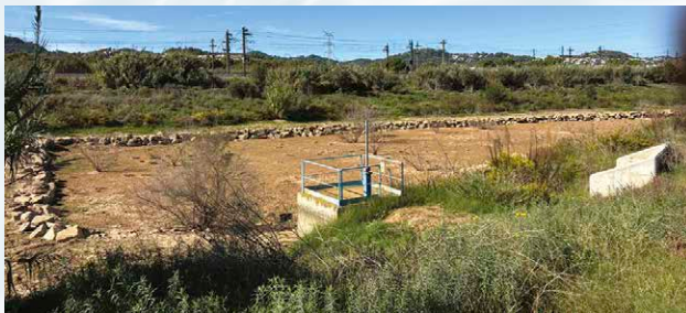
Infiltration basin along the Llobregat river.
